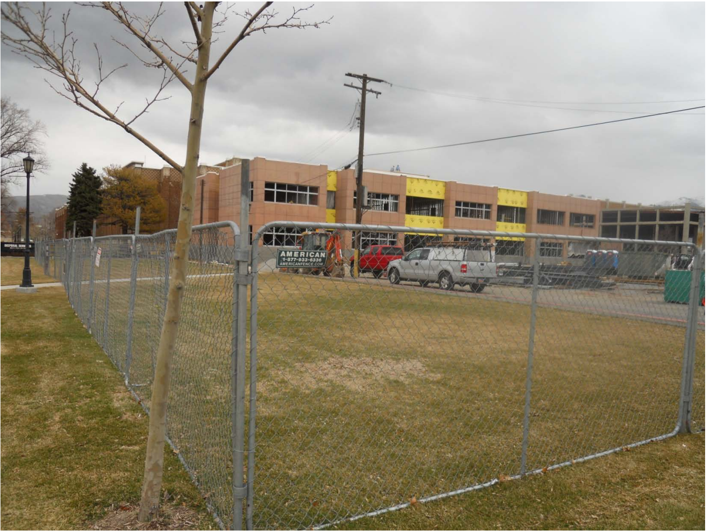
This is a southwest view of the alley proposed to be vacated.
